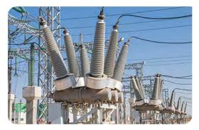
to homes and businesses world-wide. The rapid interruption of electrical power circuits is an essential function, especially in cases of overloads or short circuits when immediate current flow interruption becomes necessary. Circuit breakers perform this function repeatedly, reliably, and quickly.
